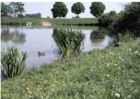
Rainwater reservoir Anecamp
