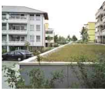
Carport with roof planting
