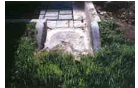
The new gulley inlet
