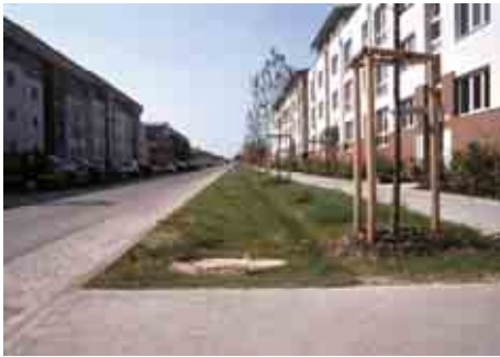
Gulleys at Ellernbuschfeld
