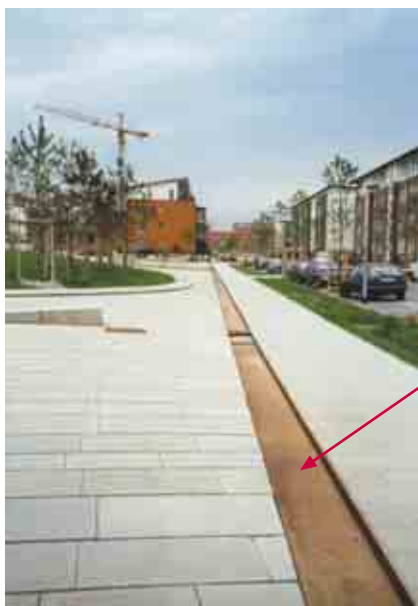
Box channel with sound opening
