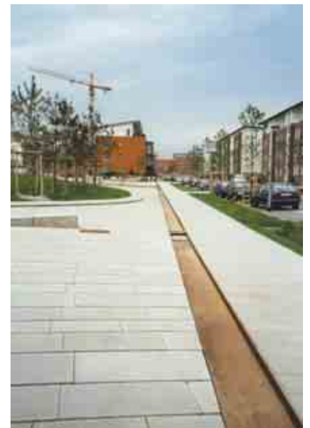
Boxed-in drain with sound opening
