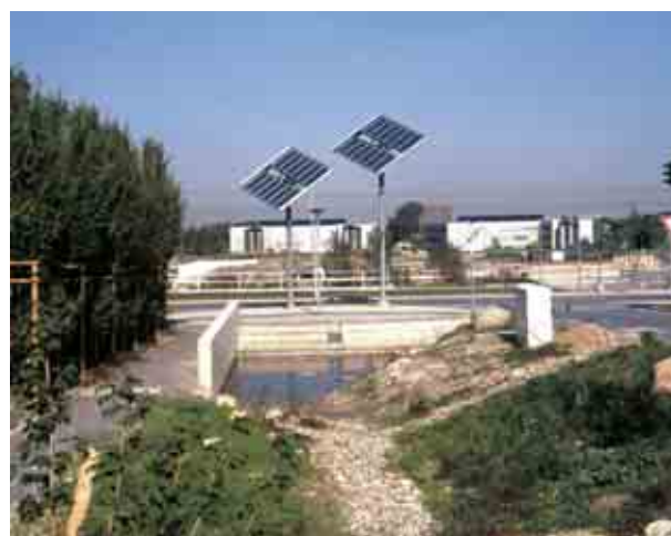
Photo-voltaic plant on the slope of Weinkampswende
