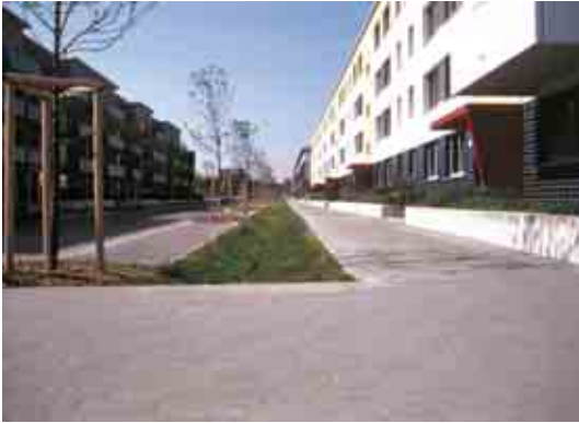
Street-laid gully and trench system
