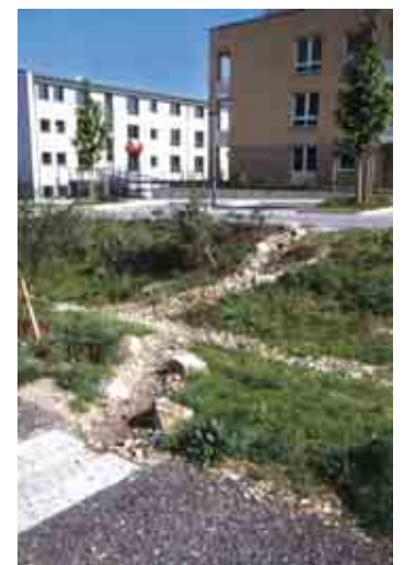
Weinkampswende - rainwater channel
