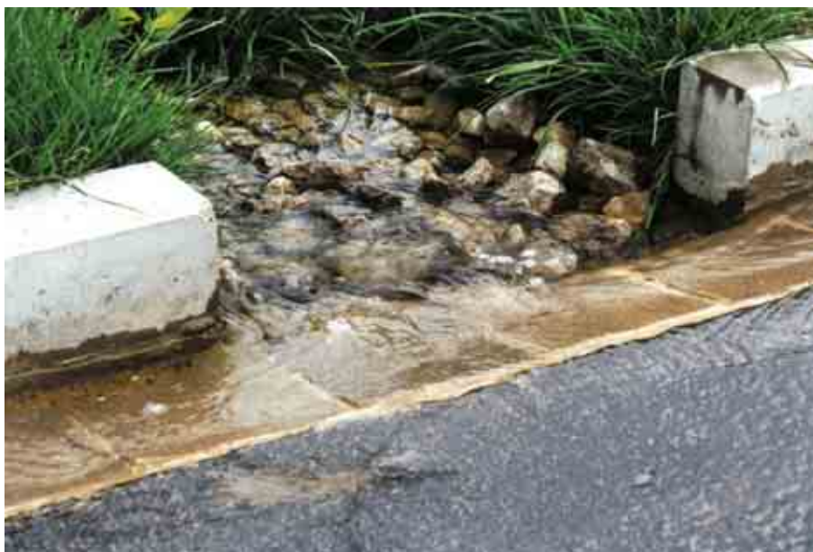
Gully lead with ballast packing
