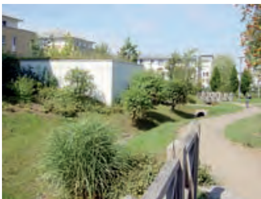
Rainwater drainage in a private inner court at Kronsberg with the 'hollow and filled trench' system
