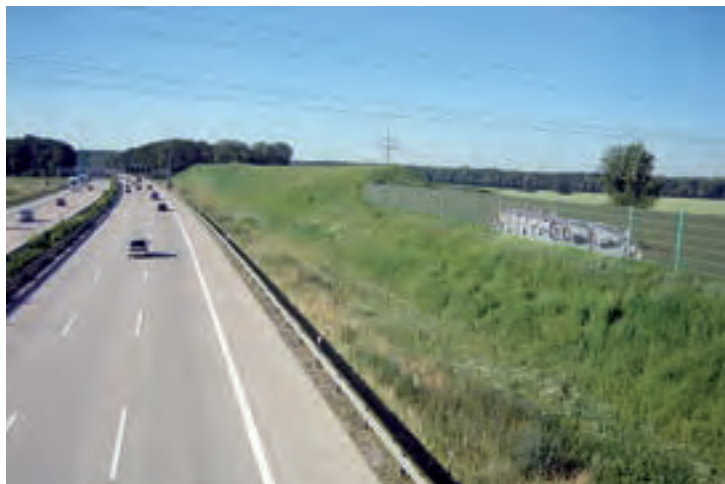
Using excavated soil to build noise buffer embankments
