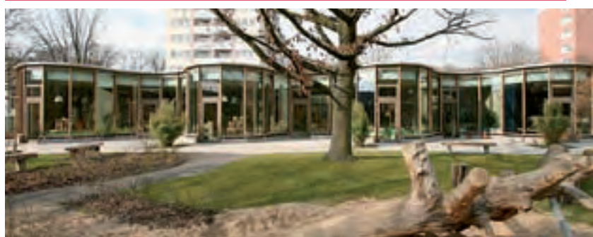
South-facing aspect – children's day centre to Passive House standard
