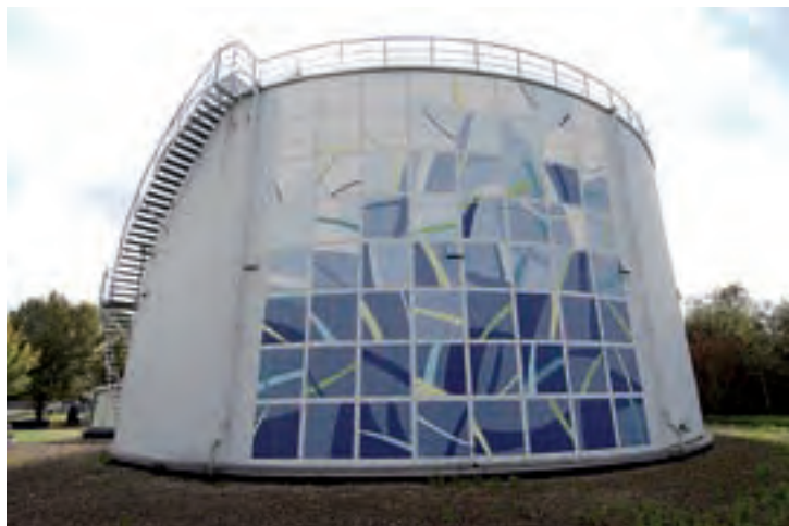
Fermentation gasholder at Herrenhausen sewage works
