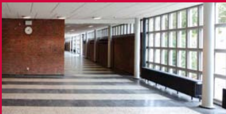
Fridjof-Nansen-School (primary school): Energy-efficient renovation with listed building conservation
