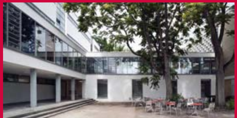
Humboldt Grammar school: energy efficient renovation of a 1960 construction.
