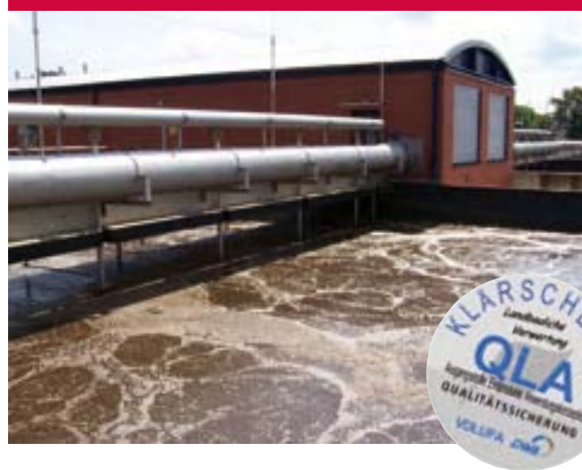
Herrenhausen sewage treatment plant
