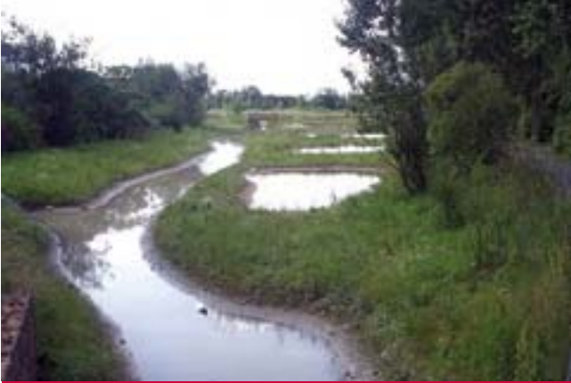
Renaturalisation of the Rohrgraben in Hannover: inundation shortly before (above) and shortly after (below)
