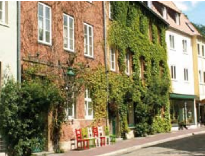
Façade greenery alleviates extreme temperatures
