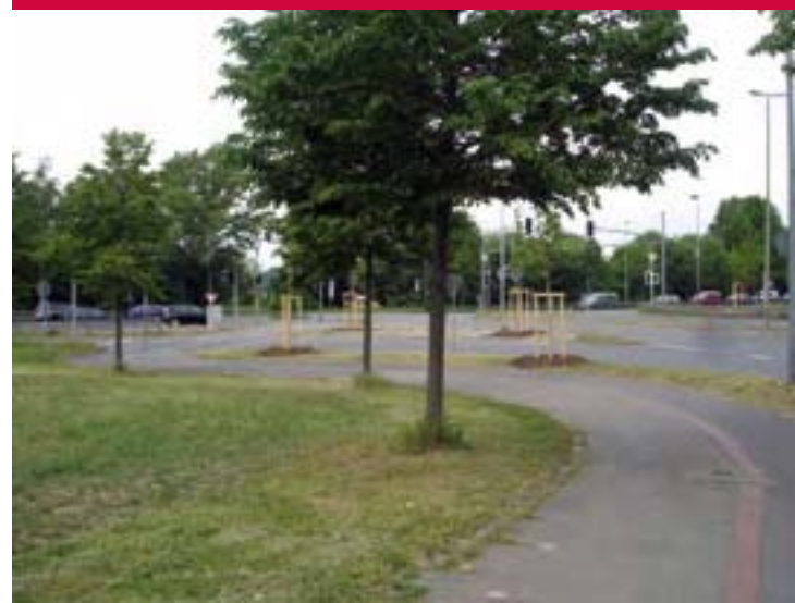
Planting of new roadside trees on the traffic island, Stöckener Straße
